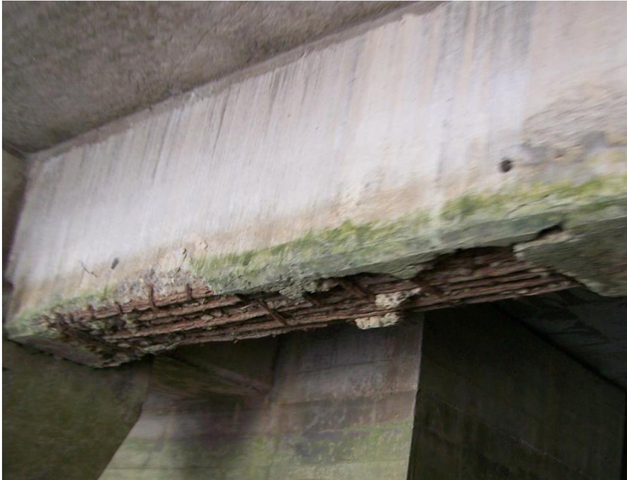
Figure 4-10: Damage of Beam [Consultant]
