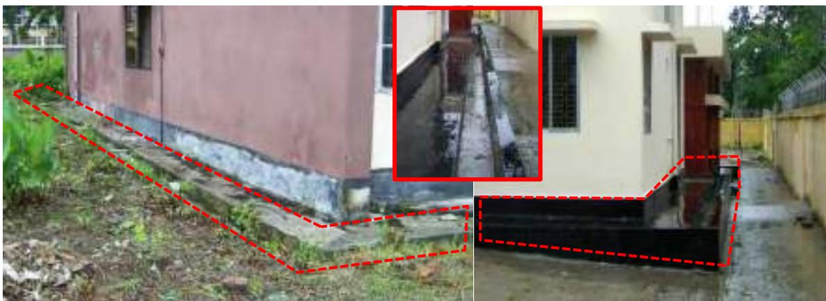
Figure 2-23: Typical Drainage Trenches around Houses [Consultant]
