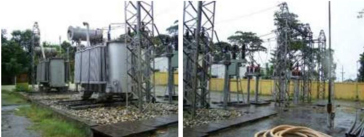
Figure 2-15: Open Transformers 33 kV / 11 kV / 415 V behind MPA Service Yard [Consultant]
