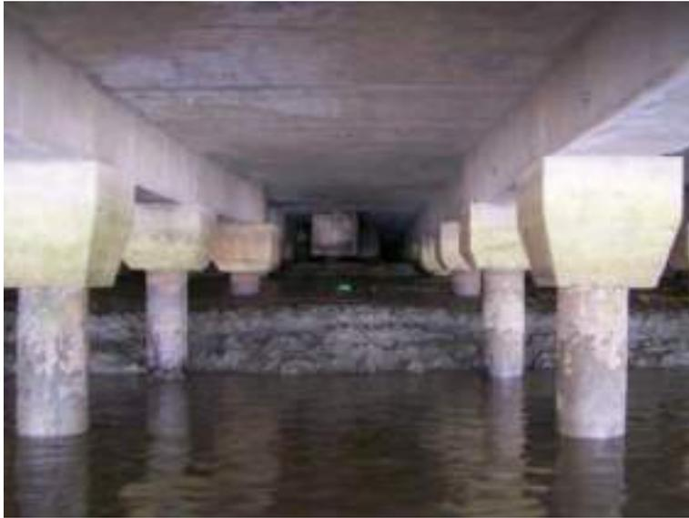
Figure 2-5: Underside of Quay Structure [Consultant]
