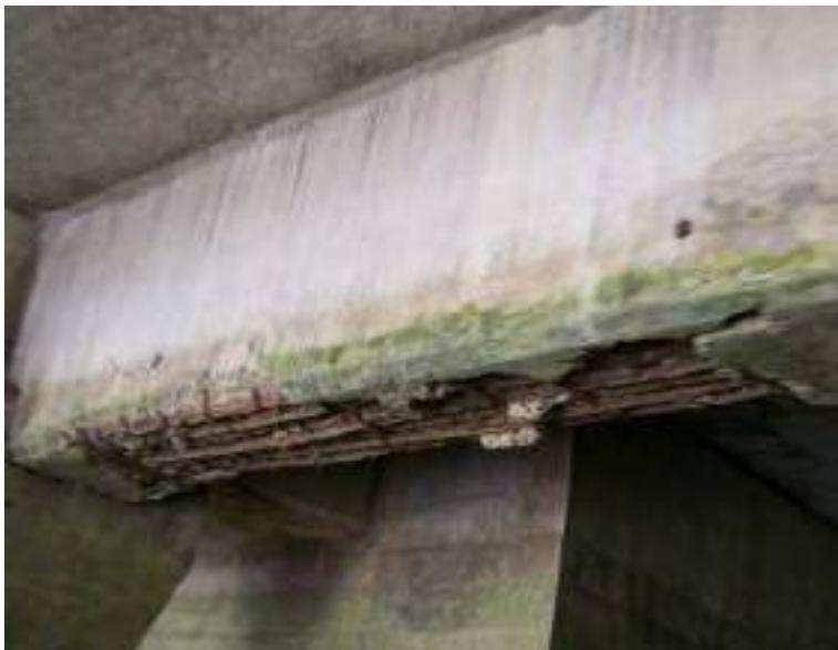
Figure 2-6: Damage of Beam [Consultant]
